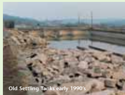
Old Settling Tanks early 1990's
