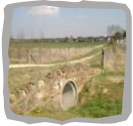
Drainage Channel Bridge (See Waymarker 4)
