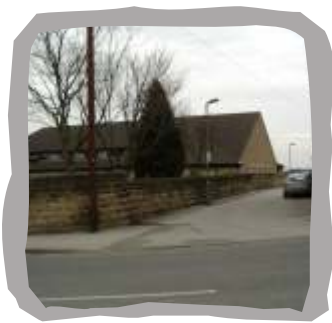
Footpath leading to Grove Terrace (See Waymarker 2)
