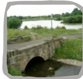
Bridge over drainage channel (See Waymarker 5)
